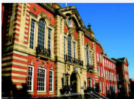
Main entrance of the St George's Building
